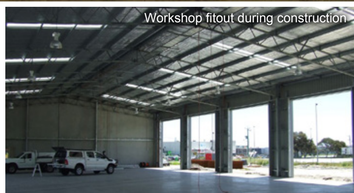
Offices during construction, workshop ready for wall sheeting
